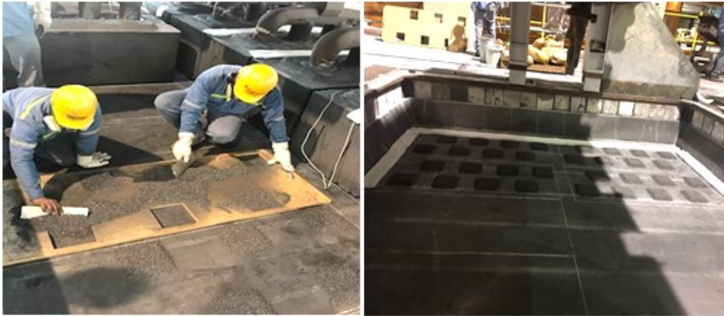
Figure 2. Surface of newly lined cathode and laying of resistor pads.
